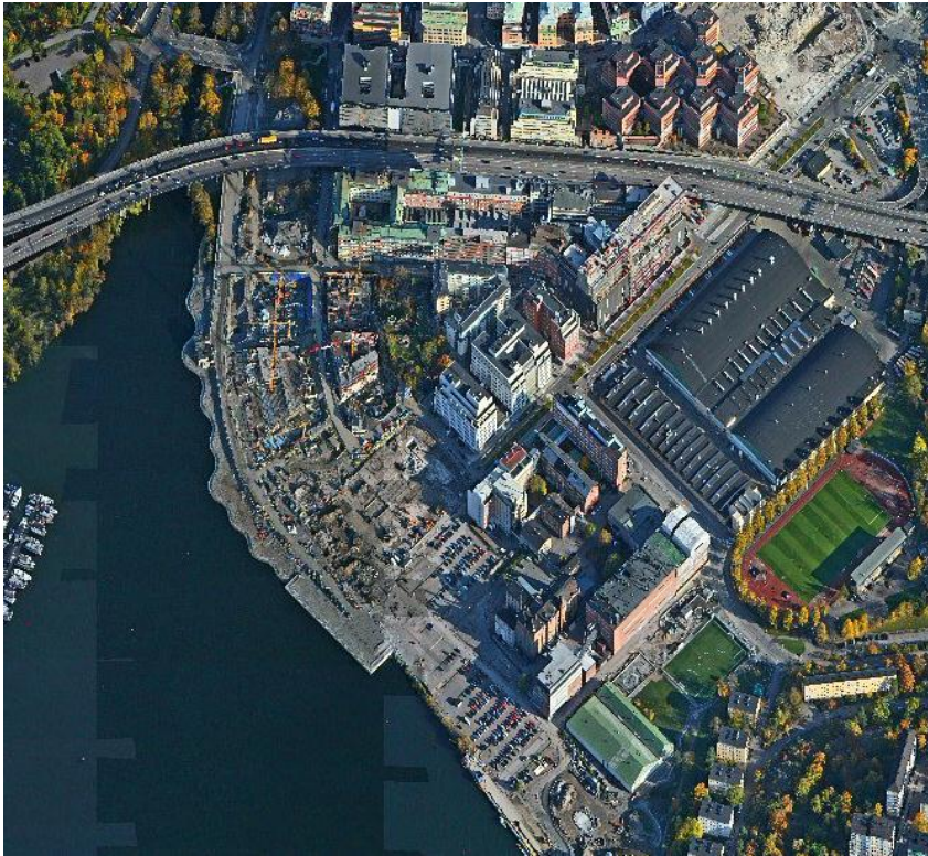
Figure 1. Overview of the project site Hornsberg Strand, Stockholm.
